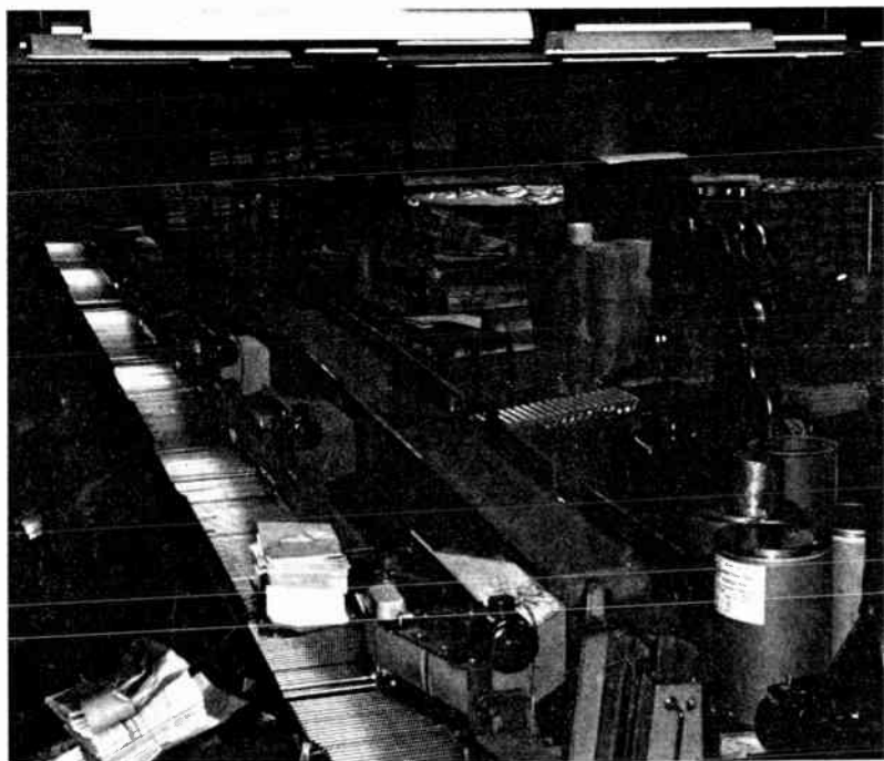
FIGURE 4. Bundled papers traveling along the mailroom conveyor system to any one of 18 preprogrammed down chutes to waiting distribution trucks.
