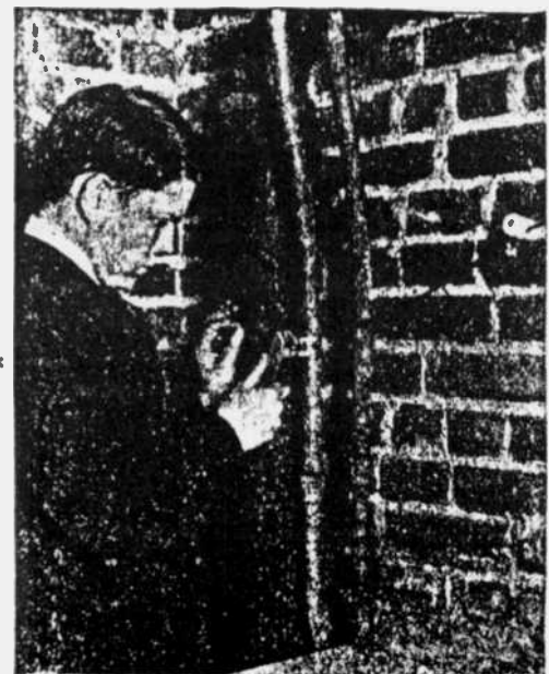
IV How the ground lead is attached to the water pipe by means of a ground clamp. Q is the ground wire.
