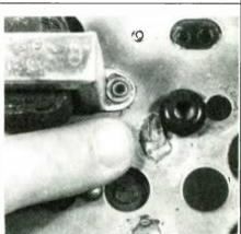
New vinyl capacitor-mounting grommets, which are much more rigid than the rubberized originals, were installed in place of the dried-out rubber ones.
