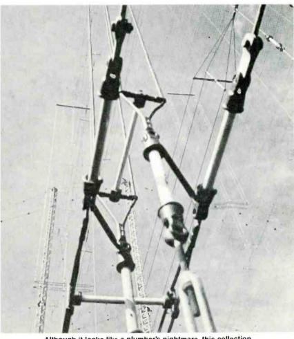
Although it looks like a plumber's nightmare, this collection of pipes, connectors, wires, and guys is really part of the curtain array station at Kigali, Rwanda in East Africa.
