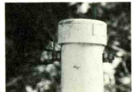
Fig. 3—Connecting the dipole segments to the mast's top terminals. Note cap to keep inside of mast dry.
