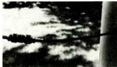
Fig. 4—Coaxial cable exits at bottom of mast. It is coupled to the lead-in line to the receiver.
