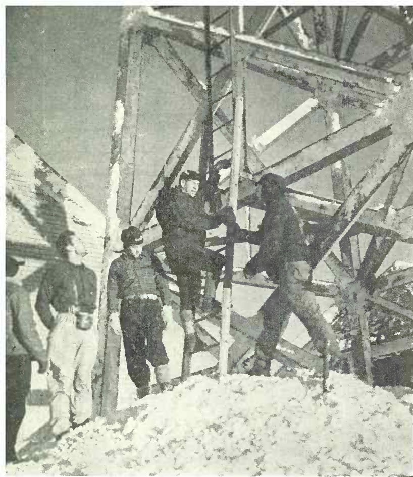
WINTER CREW preparing to inspect Mt. Washington FM tower.
