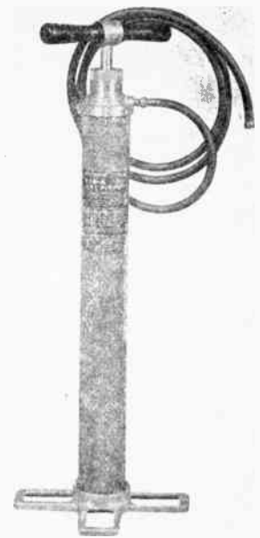
FIG. 25B. MANUALLY-OPERATED DRY AIR PUMP FOR COAXIAL LINES
