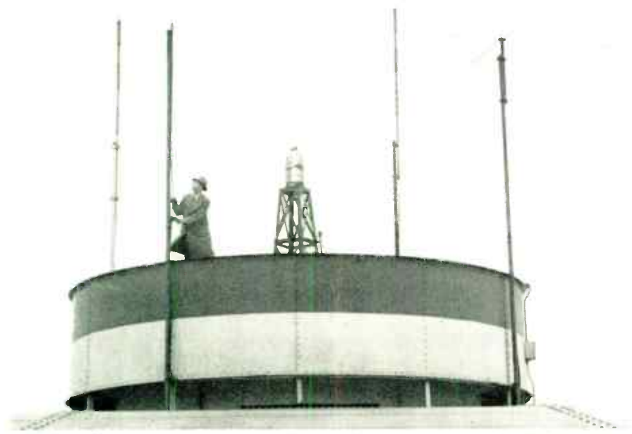
FIG. 2. Technical Sergeant Severin Barstad checks the antennas atop the gas holder
