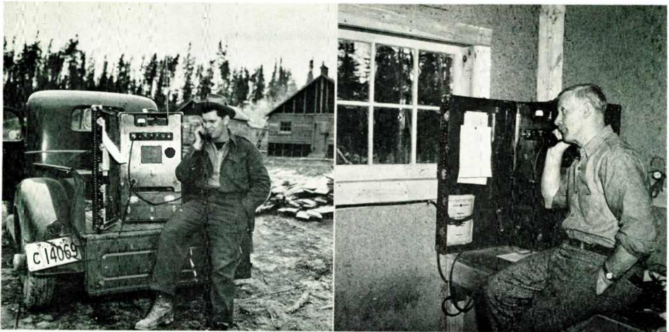
FIG. 5. ENGINEER SНИЕZEK USES TRUCK DURING CAMP CONSTRUCTION. FIG. 6. BOSS WHITE'S OPERATING SHACK AT CEDAR LAKE
