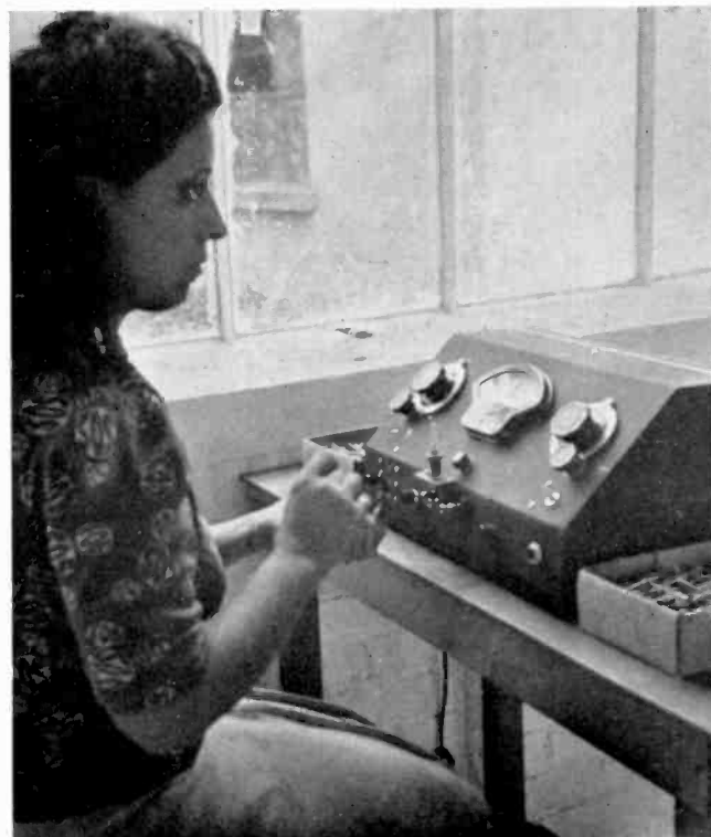
FIG. 1. CHECKING CORES ON PRODUCTION TYPE Q METER
