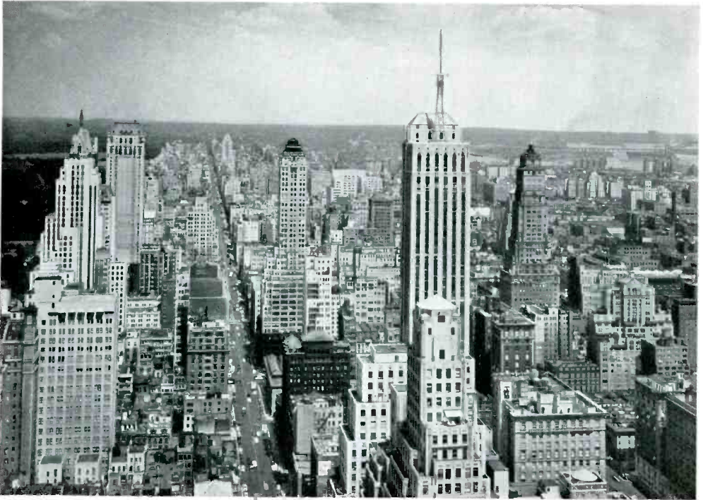
DU MONT TELEVISION TRANSMITTER W2XWV, AT 515 MADISON AVENUE, NEW YORK CITY
