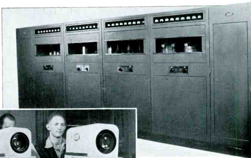
ABOVE: VIDEO AND AUDIO TRANSMITTERS INSTALLED AT TELEVISION STATION W2XWV
