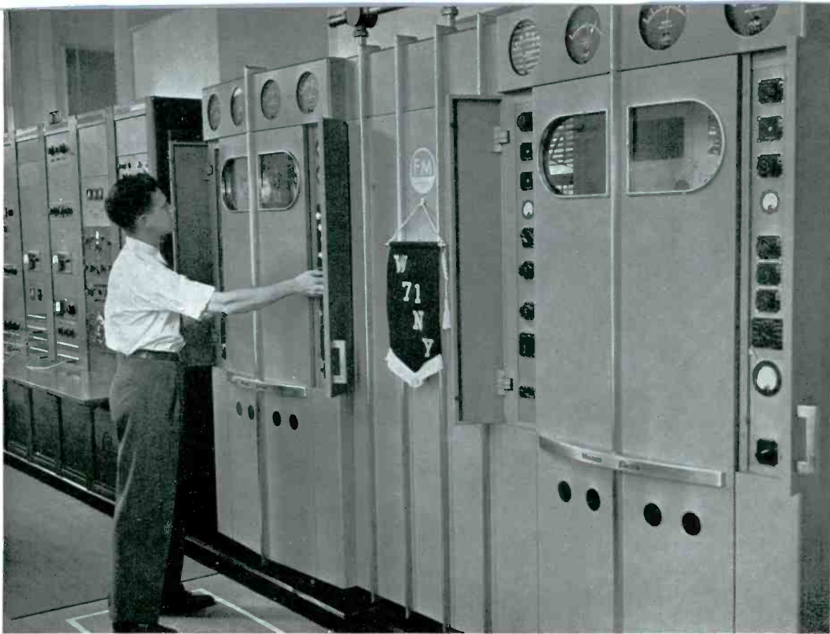
FIG. 1. W71NY HAS THE FIRST WESTERN ELECTRIC 10-KW. FM TRANSMITTER TO BE DELIVERED
