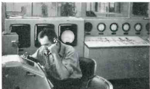
Simultaneous transmission of numerous telemetering and voice signals over one radio-frequency carrier allows positive, instantaneous control over widely separated, remote system facilities.
