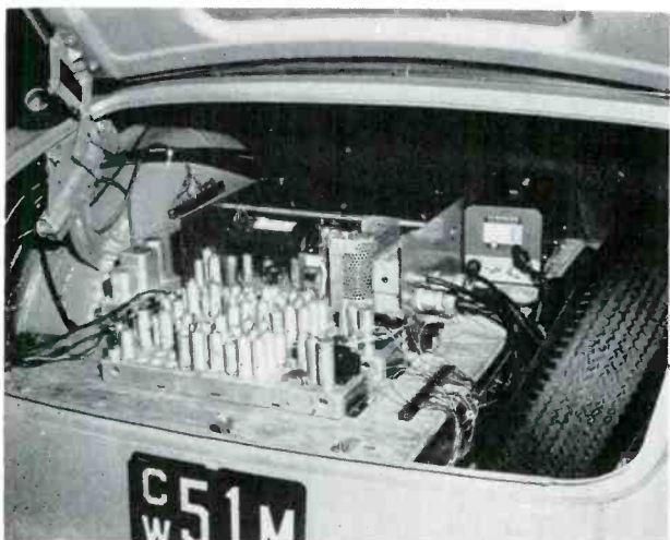
FIGS. 12 AND 13. THE 60, 30, AND 20-KC. RECEIVERS MOUNTED IN TEST CAR LUGGAGE COMPARTMENT, AND THE INSTANTANEOUS SWITCHING CONTROLS
