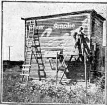
The walls were covered with tar paper
