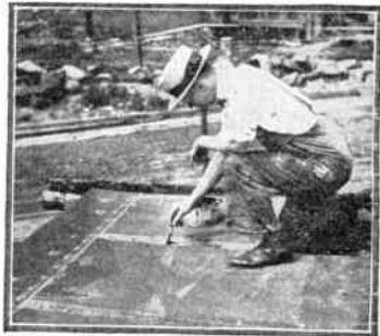
The seams in the tar paper were painted with asphaltum
