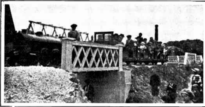
Engine and train passing over bridge on Margate miniature line that spans a roadway
