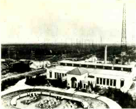
Photo shows the Rocky Point transmitting station with its swimming-pool that provided cooling water for the transmitters. Behind are a few of the 12, 410-foot tall long wave antenna towers.
