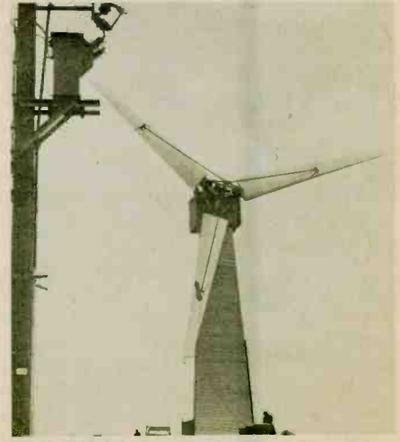
On the pole to the upper left of the windmill you can see the special installation which receives the grid-synchronous portion of the generated power. Once into the main power-network it can be directed to wherever it may be needed.
