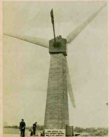
The aerogenerator uses standard components such as fixed blades instead of variable-pitch ones. Even though it rotates, due to the fixed blades, at a constantly varying speed, a complex hydraulic system ensures the generators turn steadily.
