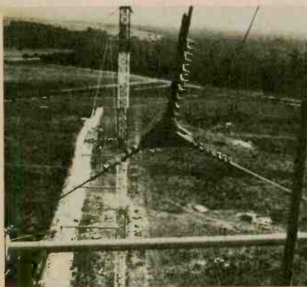
View from the top of a curtain antenna which comprises part of the Deutsche Welle's Sines relay station in Portugal.
