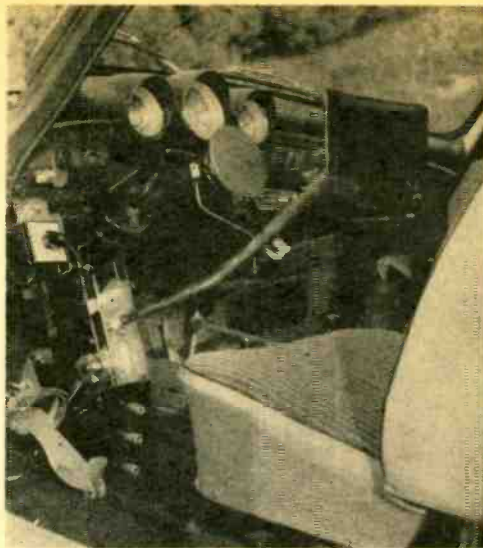
Photos show some of the modifications in Mr. Franz's car. At top, column replacing steering wheel is chest pad for activating power breaks. Below, left foot is on steering device. Note starter lever next to left knee.
