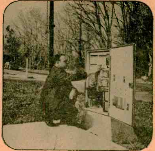
This roadside computer (above) feeds directions to drivers hooked-up to ERGS who then receive clear, bright signals on the electronic indicator (left) installed on the dashboard of their car.
