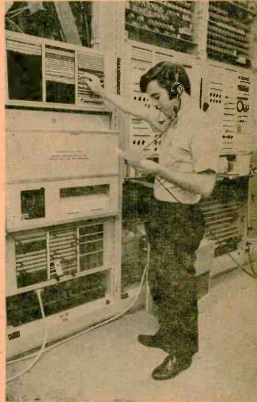
This computerized monitoring board known as MOM (above) punches out a computer card at the central office from a high-speed tracer which is attached to your home telephone.
