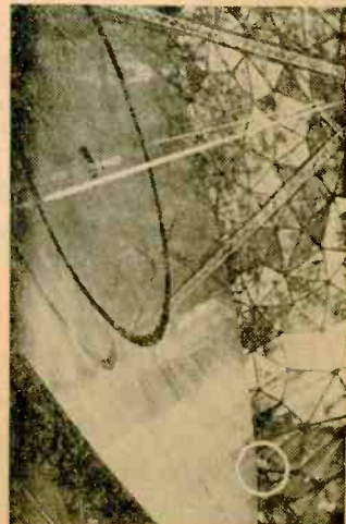
Installation at Haystack Microwave Research Facility (operated by M.I.T.'s Lincoln Laboratory for U.S. Air Force) boasts 120-ft antenna within 150-ft diam radome. Note man within circle in closeup at right.
