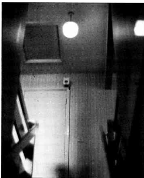
Fig. 1. Correct position of smoke detector.
