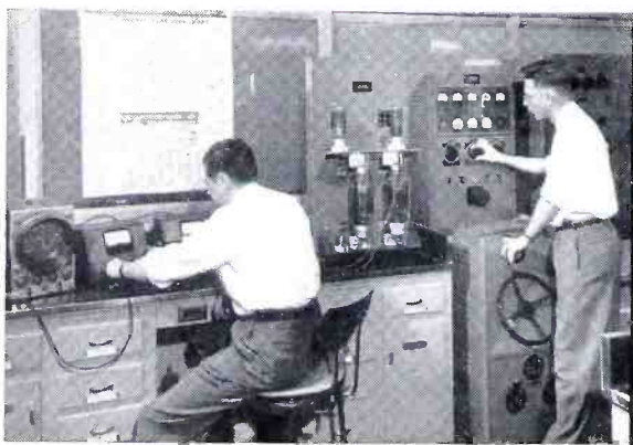
Testing modulation transformer under operating conditions
