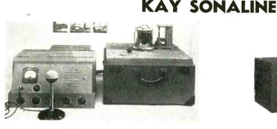
**SONA-GRAPH** A fourier analyzer for complex audio waves. Frequency range: 85-8000 ps. Recording time: 2.4 seconds. Amplitude display: 35 db. Price \$1595.
