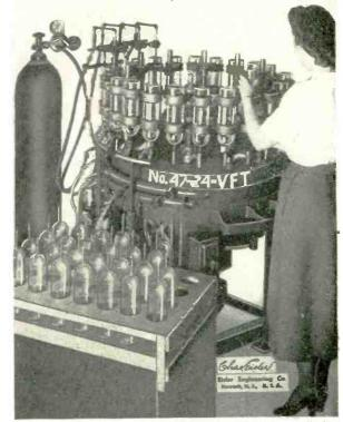
Automatic Piercing and tubulating machine for vacuum flasks.
