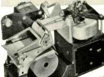
with extremely high torque movement (200,000 dyne cms), ruggedly built and producing clear, permanent records.
