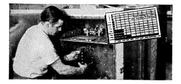
**Insulation Resistance Test on Various Grades of Dilecto** —This is one of several test procedures necessary to evaluate an insulating material, and for classifying various types and grades of such material. The test serves also to establish the relative uniformity of the material.
