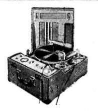
K8 Recorder (12") is complete with amplifier and speaker, operates at both 78 and 33½ rpm, outside-in and inside-out. It is equipped with a high frequency equalizer. Fifteen minutes of voice quality may be recorded on a single side of a 131/4" disc. This unit is used by many schools, colleges, broadcast stations and recording studios.
