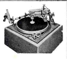
8N Recorder (16") is well known to broadcast and recording engineers. It is a rim driven unit employing a heavy cast iron turntable and an overhead mechanism of unusually solid construction which is driven from the center of the turntable. Change of feed pitch and direction is accomplished by changing feed screws.
