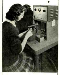
(Bench welder MODEL # 2000-56 in operation at one of the largest instrument manufacturers —THE FOXBORO CO.)
