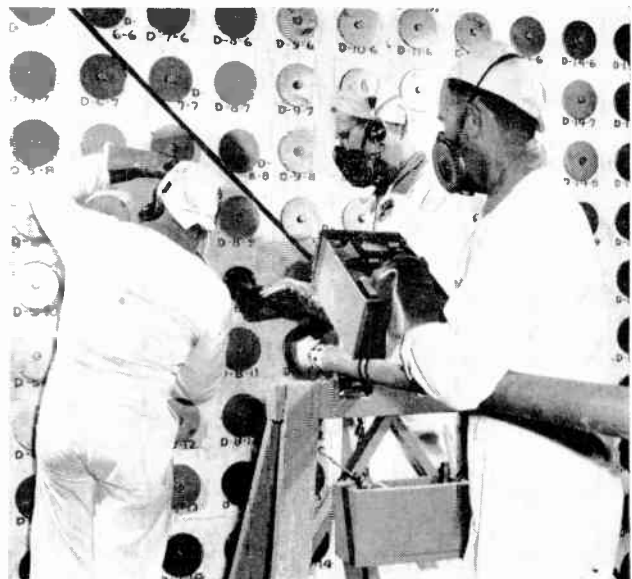
Removing spent fuel from reactor
