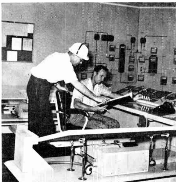
Data logger (front), indicators tell what's happening
