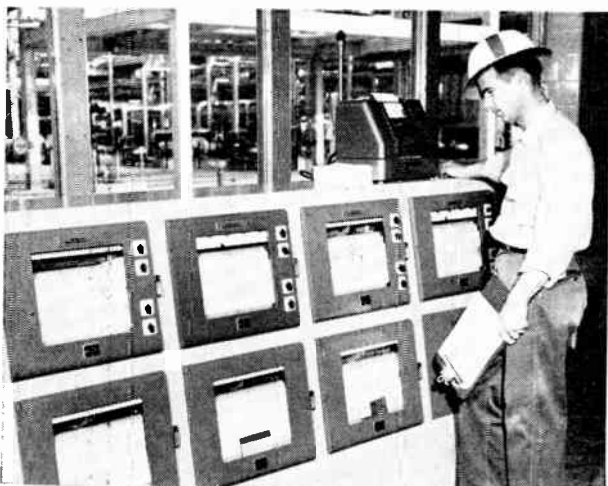
Process variables are compared on trend recorders
