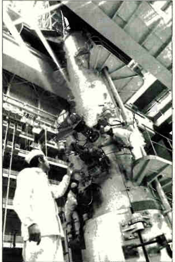
INSIDE CHERNOBYL. Workers at the Soviet nuclear plant, in the Ukraine, are carrying out maintenance on a reactor.
