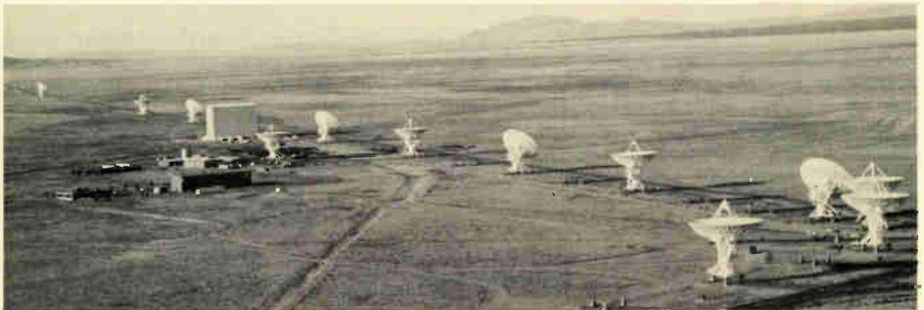
Listening. Twenty-seven of these 82-foot-diameter dishes will form the gargantuan antenna of the National Radio Astronomy Observatory's radio telescope, being built near Socorro, N. M., which uses custom-designed ECL and TTL parts.
