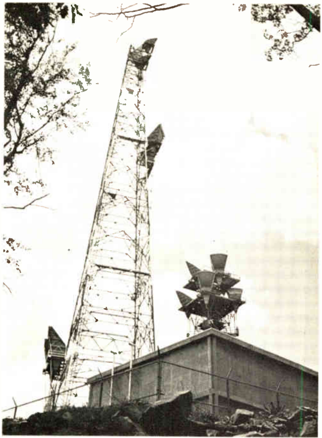
4. Saturated. Microwave relay routes in the 4- and 6-GHz bands are saturated in urban centers such as New York and Los Angeles, forcing the move to 11-GHz frequencies and higher. The use of low-sidelobe antennas and space-diversity backup systems would increase spectrum utilization efficiency at all frequencies.
