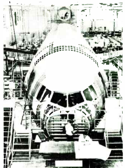
Grounded. Test system for DC-10 uses 150 hydraulic jacks and battery of computers to "fly" craft equivalent of 2,600 around-the-world trips in Long Beach, Calif.
