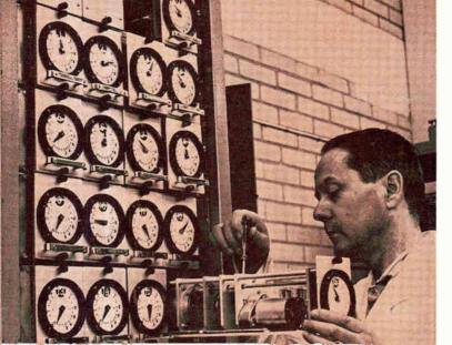
**Readouts.** Swedish electronics firms increase the penetration of the European market with specialized hardware. The race track totalizer display at left is by Swedish Computer, a part of AB Arenco. Technicians (right) test a printing device headed for bank installations at Philips Terminal system, organized after Philips acquired Arenco.
