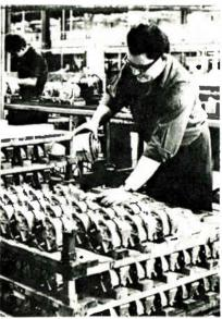
Inputs. Bosch is now mass producing alternators with IC voltage regulators.
