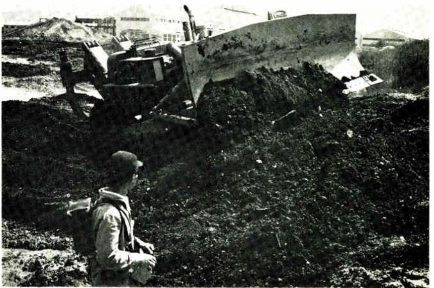
Sideline. Unskilled operator fiddling with joysticks can put bulldozer through its paces like a veteran cat skinner.
