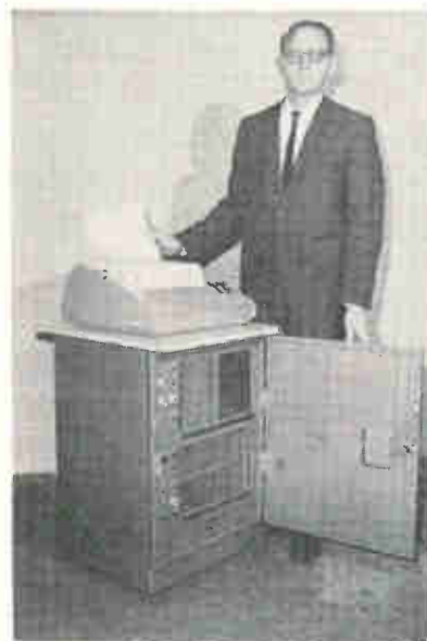
Self-contained. Basic event recorder package scans up to 250 points, types data on teleprinter.
