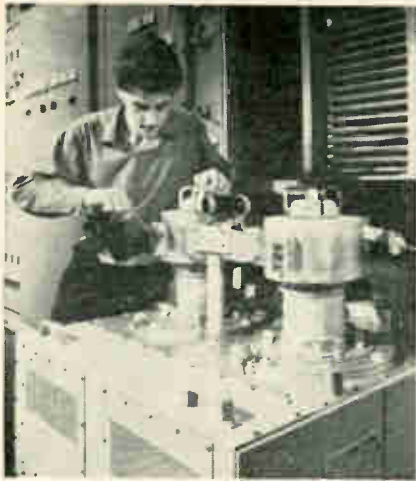
Long-wave transmitter. Two big air-cooled tetrodes provide the final amplification in new 100 kw transmitter.
