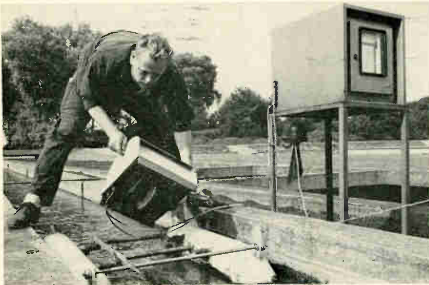
Immersed. Oil contamination in conduit of water-treatment plants is detected by drop in conductivity across electrode pairs mounted on wheel that spins with its rim dipped.
