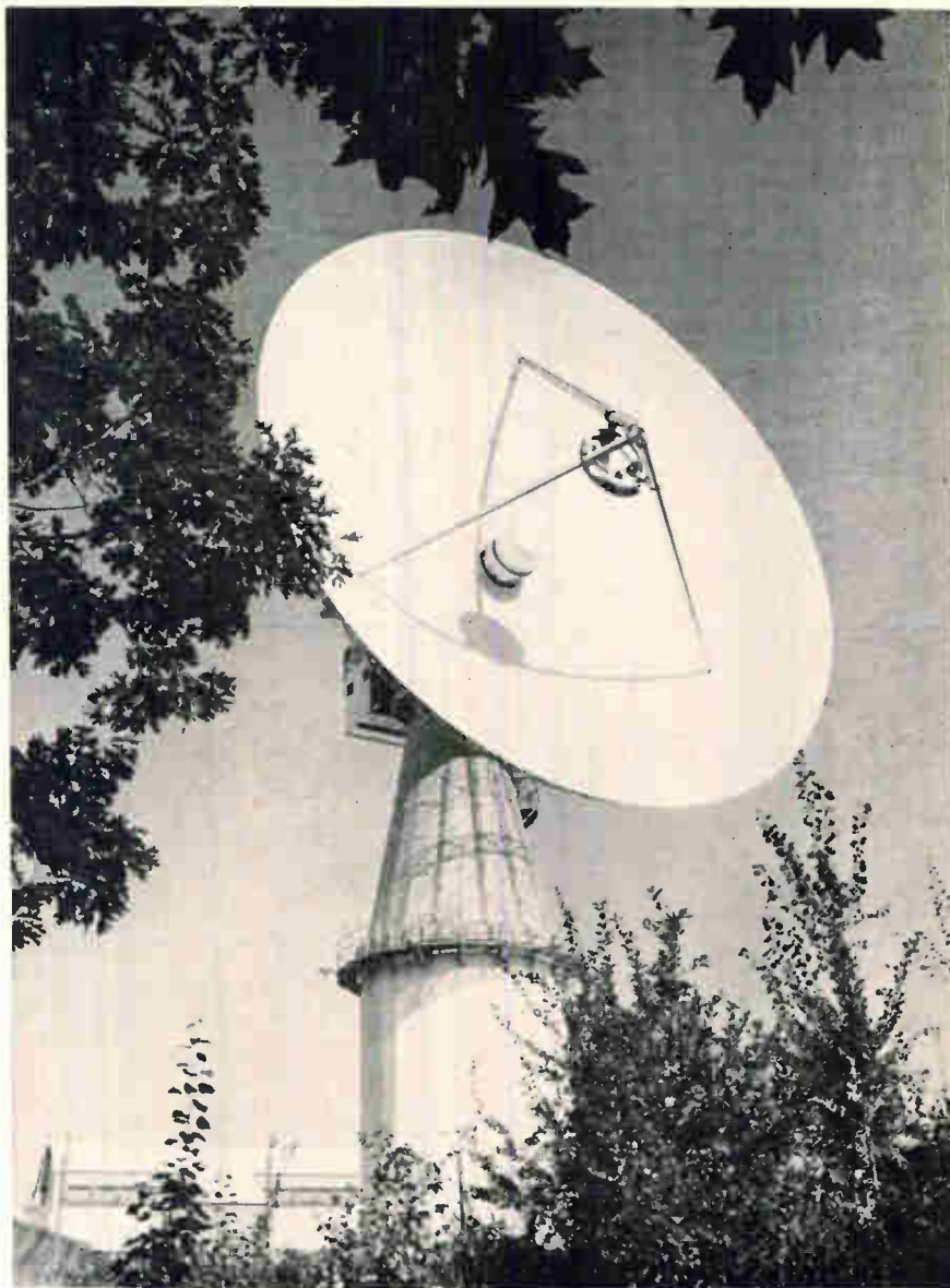
Millstone Hill radar antenna, measuring 84 feet in diameter, is key part of interferometer. MIT's Lincoln Laboratory operates the facility.
