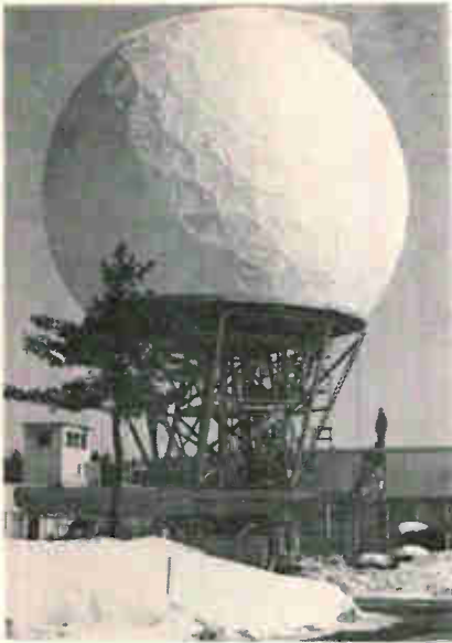
Under cover. Antenna at Mitre Corp.'s Bedford site now sports a radome.
