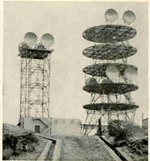
Microwave repeater stations, like this one at Futago Yama, dot the hilltops of the Japanese countryside. Inside the building is a heterodyne repeater.
