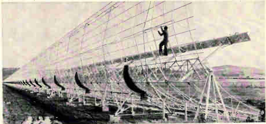
Antenna wire mesh of the mile-long east-west arm being inspected. Dark horizontal line just above ground is a motor-driven shaft that rotates the arm as much as 55° about its long axis.
