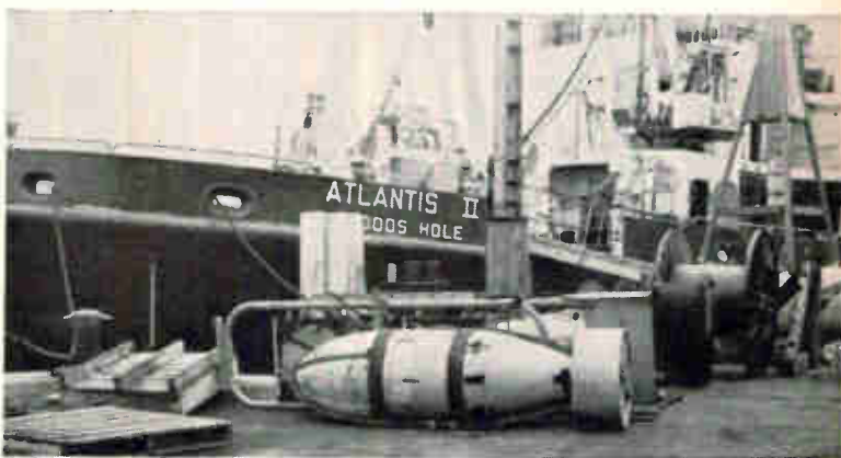
Transducer for boomer sonar ready for loading aboard the Atlantis II as she is fitted out for a cruise to Puerto Rico.
