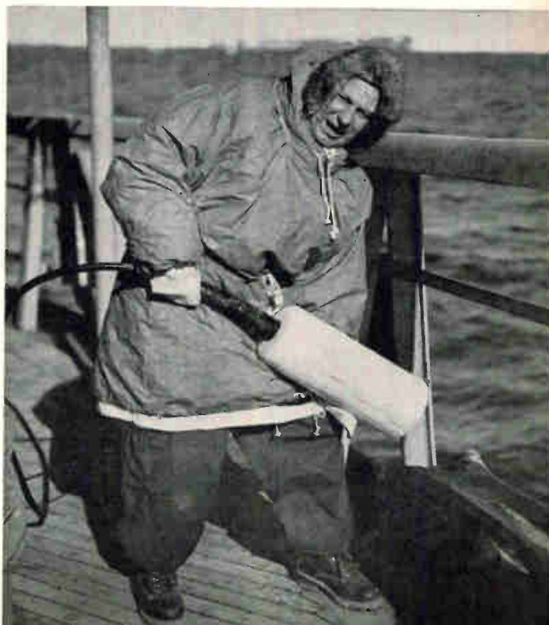
Transducer for boomer sonar ready for loading aboard the Atlantis II as she is fitted out for a cruise to Puerto Rico.
