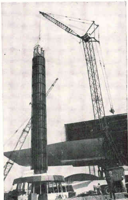
Television link between the fair and Manhattan, a single-horn antenna is being erected on a 130-foot tower next to the floating wing of the Bell System pavilion.
