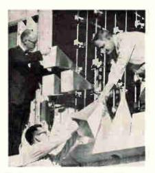
Putting bigger horns on the little horn radiators improves concentration of the radiated r-f power
