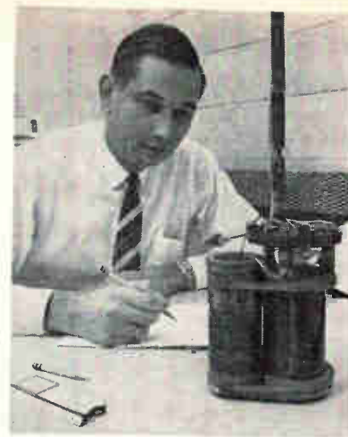
COMPACT 375-joule energy source developed by Ion Physics. A 50-liter coil, including dewar, can store 100 joules, while capacitor banks require 750-liter volume for the same job
