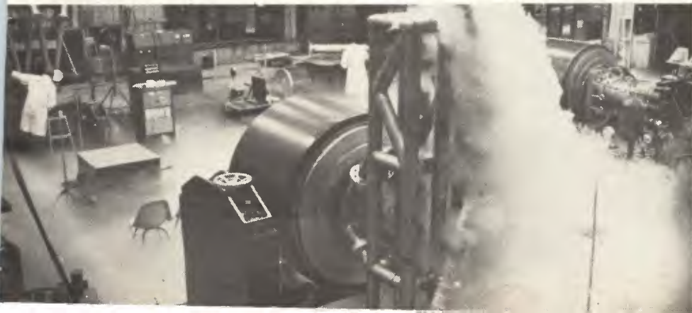
LTV Ling Electronics Division's powerful L-200 shaker vibrates Saturn S-IV rocket components.
