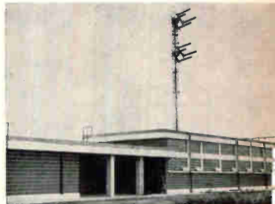
STATION built in the State of Mexico for the microwave system and to handle international Telex traffic via RCA Communications
