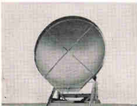
■ 20 meter diameter antenna for satellite communication
