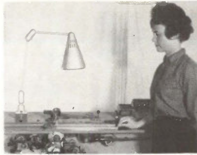
RESISTORS in rack are each automatically printed with serial number, trademark, type number, value and date
