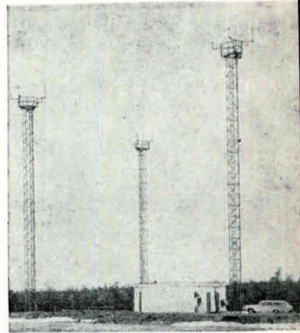
REMOTE SITES pick up voice messages (vhf and uhf) from pilots and relay them by land line to distant centers below the horizon
