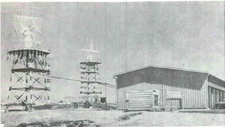
ROUGHING IT at Muchea. This is the telemetry and control facility at the Mercury tracking station
