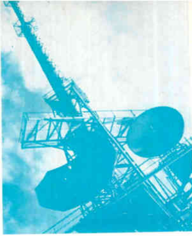
TELEVISION TRANSMITTER in Austria will radiate German language programs to four and a half million tv screens. Telefunken engineers erected equipment, Austrian, Swiss and German engineers will operate it
